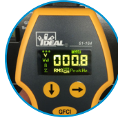
Displays neutral to ground voltage
