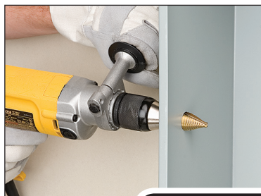
Drill Pilot Hole
