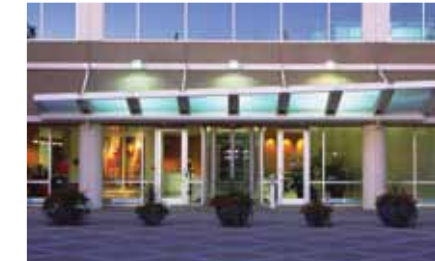
outdoor facility lighting
