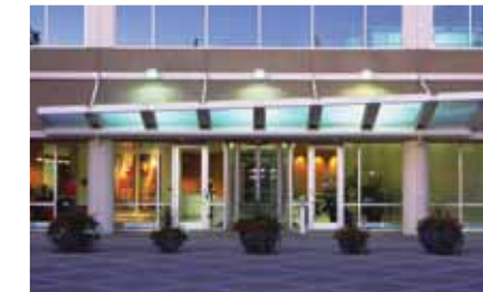
outdoor facility lighting
